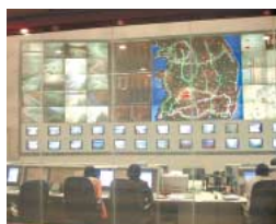
Traffic control center
